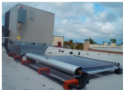
Example of March 2011 Installation of Sedna Aire Solar Air Conditioning System which included the SOLAR COOL Logo.
